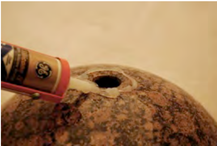
Caulking location for Stone Vessel Sink
