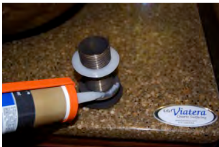
Caulking location for Stone Vessel Sink
