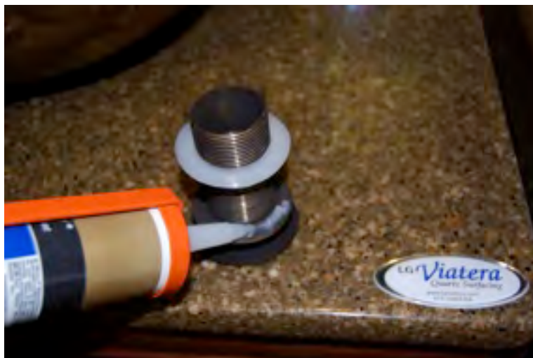
Caulking location for Stone Vessel Sink
