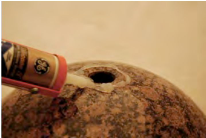
Caulking location for Stone Vessel Sink
